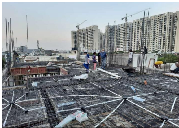
Inspection before Casting of Slab at Sec-22, Gurgaon
