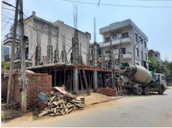
Residential building Concreting Work in Progress at sec-54,Gurgaon
